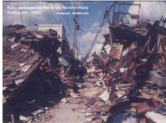
Photo 2: Collapsed houses in Kobe
