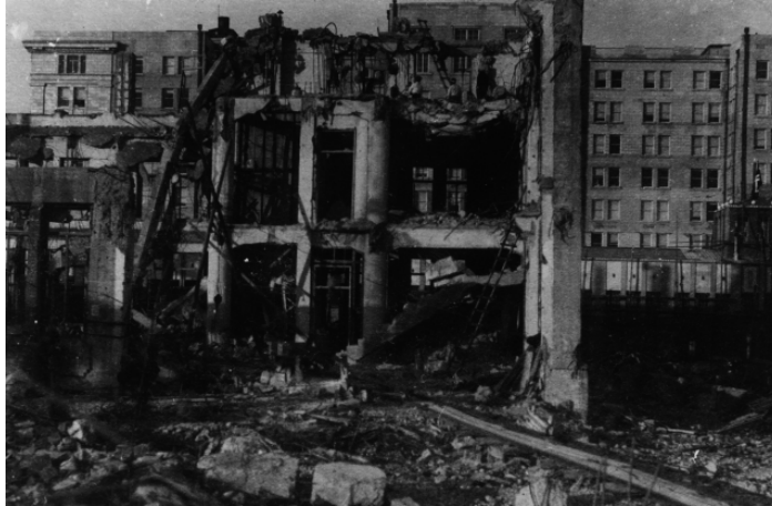
Photo 2: The Naigai Building near completion collapsed
