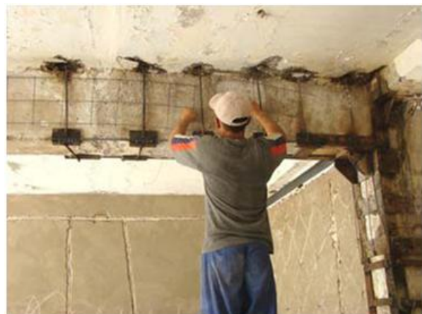
Fig. 7 Retrofit of RC panel school in Tashkent (UNCRD).
