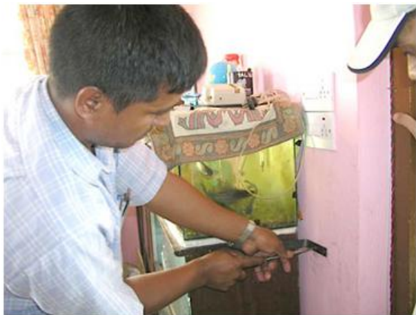
Fig. 5 A trainer of NSET secures furniture using anchors in a community participant's home in Kathmandu (by UNCRD).
