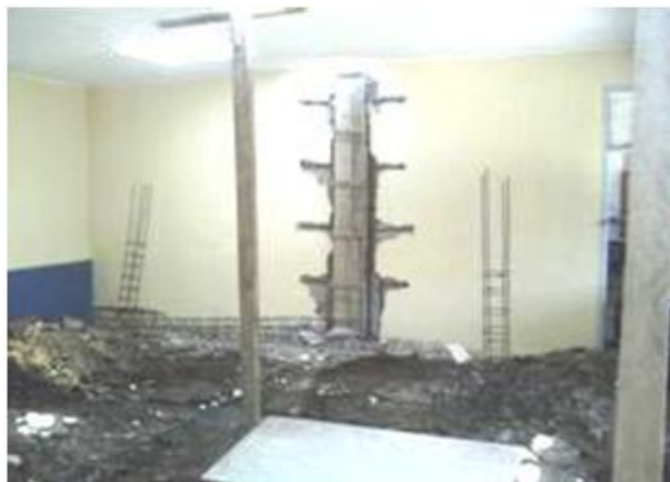
Fig. 6 Retrofit work of School Building I (ITB ).
