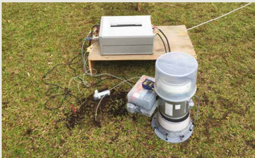
The monitoring device is being tested in the field
