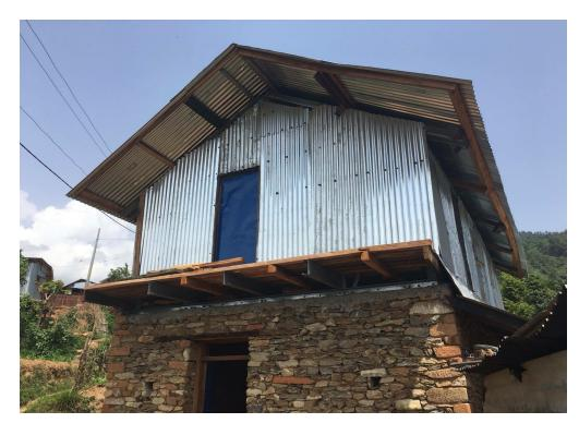
Figure 2. Rebuilt earthquakeresistant two-story local house.
