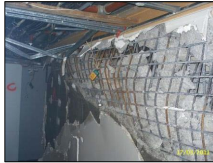
(f) Diagonal crushing of web concrete region; Terrace on the Park (2000-2010)
