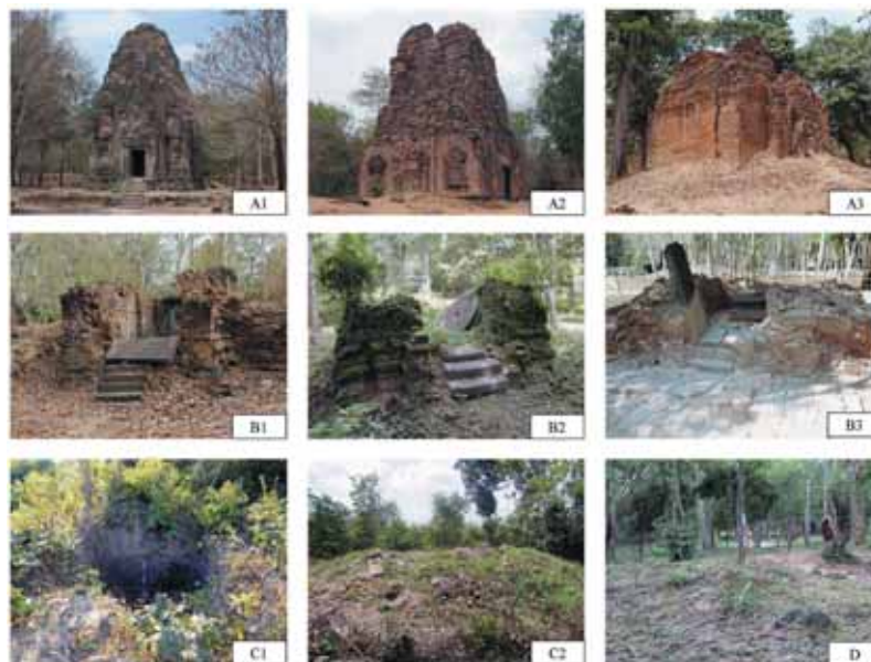
Figure 5. Classification of the state of preservation (A1: S1 shrine in Prasat Yeai Poeun (M.24), A2: N15 shrine in Prasat Sambor (M.20), A3: N13 shrine in Prasat Sambor (M.20), B1: S6 gate in Prasat Yeai Poeun (M.24), B2: S17-1 shrine in Prasat Yeai Poeun (M.24), B3: N14-2 shrine in Prasat Sambor (M.20), C1: brick structure at M66-1, C2: brick structure at M68, D: C19-1 brick structure in Prasat Tao (M.26)).
