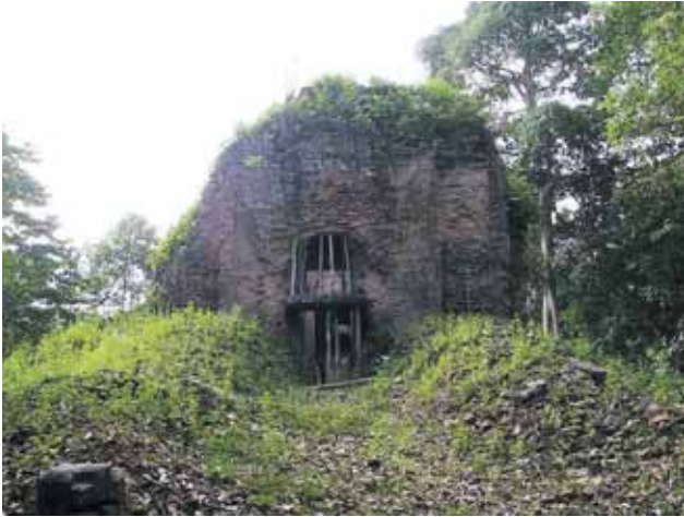
Figure 14. North elevation of the Central Shrine in Prasat Sambor, before restoration.
