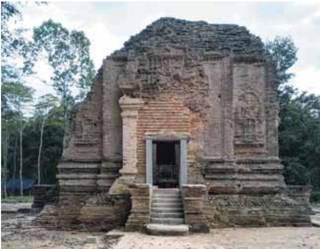
Figure 15. North elevation of the Central Shrine in Prasat Sambor, after restoration.
