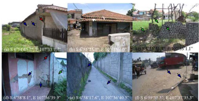
Fig. 4. Sample photographs collected during a ground survey conducted on December 13–14, 2008, February 25–28, 2009, and August 4–10, 2009. Serious land subsidence affected the Cimahi, Dayeuhkolot, and Baleendah industrial complexes (IC1, IC4, and IC5). Cracked walls and roads were observed in residential, irrigation, and industrial infrastructures. The red, green, and blue arrows indicate vertical, diagonal, and horizontal cracking.
