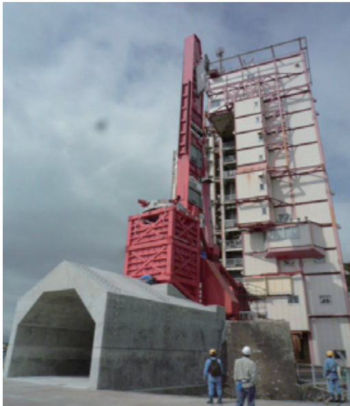
Fig. 10. The modified launch facility to lower the level of acoustic environment at launch.
