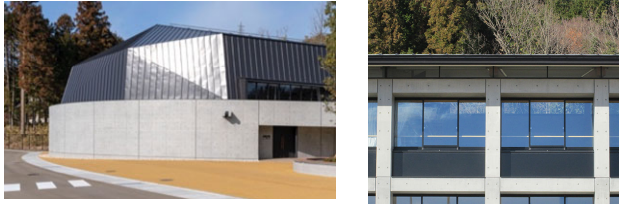
Fig.6 Solar Collecting Roof / Wall
