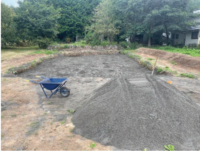
Figure 4: Suwahara site after excavation. The site was protected with sandbags placed in trenches and pits, covered in two blue tarps, and filled with sand. (26 September 2021)
